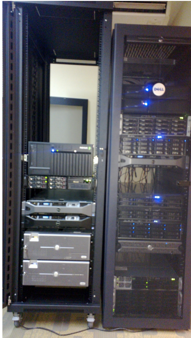
Figure 4.12: Machines' storage facility, located in DCC.
